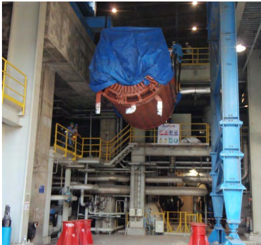
NPS- Thatoom Alstom Stators Swap Thailand
